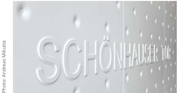
Effectively animated outside, inside a clear design of dots and letters milled out by using the CNC technology.
